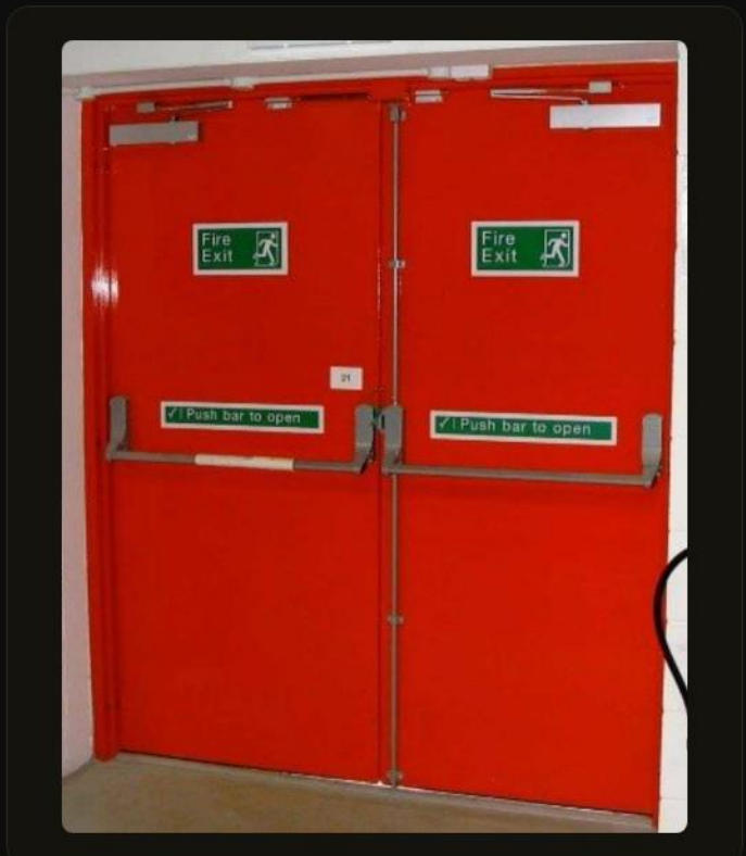
Steel fire-rated exit doors · push-bar exit hardware
