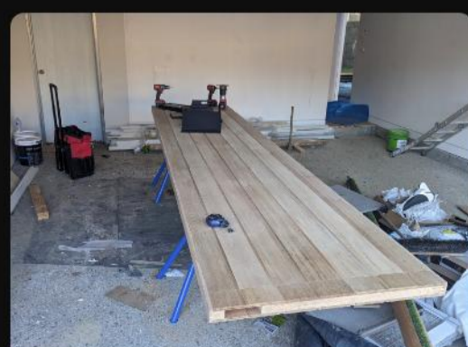
Glen Waverley · 4m oversized, structural reframe
